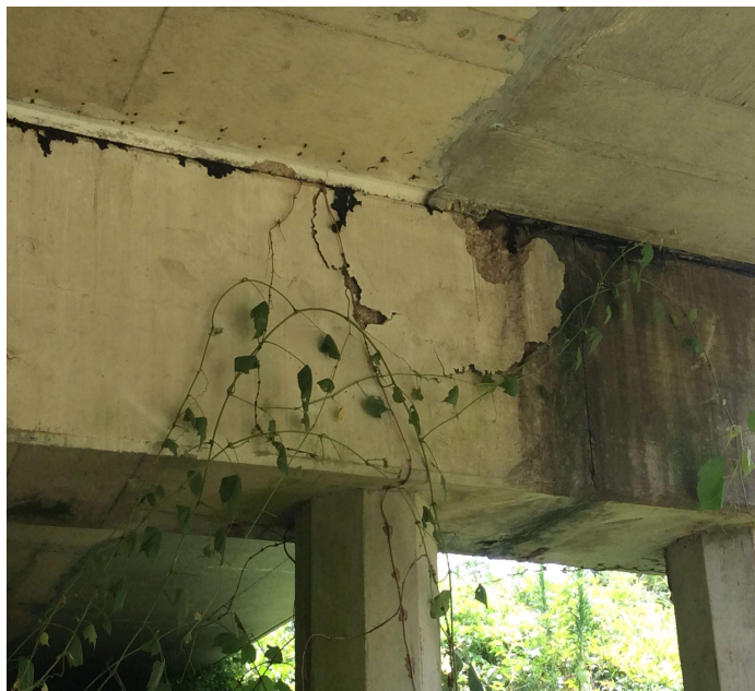
PHOTO 27 Description Bent 25 spalls and delamns.
