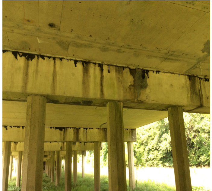
PHOTO 9 Description BT 10 spalls rebar exposed and delam 9 total LF . 6 LF rebar 3 LF delam
