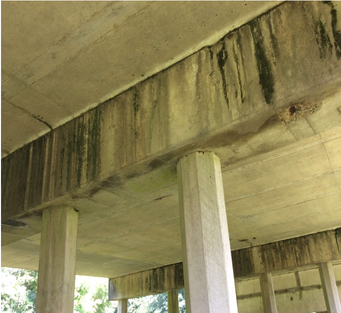
PHOTO 7 Description BT 13 spall with rebar exposed and delam Spall rebar 3 LF
