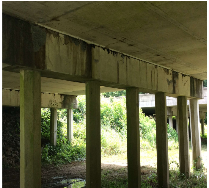
PHOTO 26 Description Bent 24 spalls and delamns.
