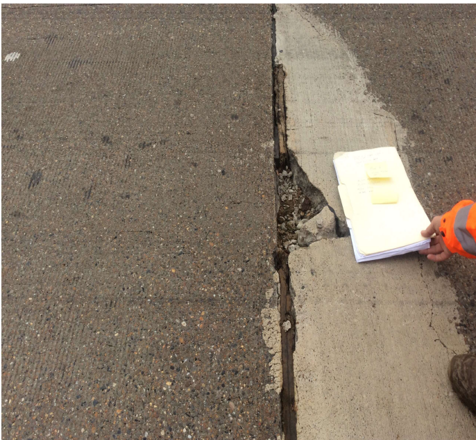
PHOTO 1 Description HOLE IN DECK BENT 21 SLOW LANE
