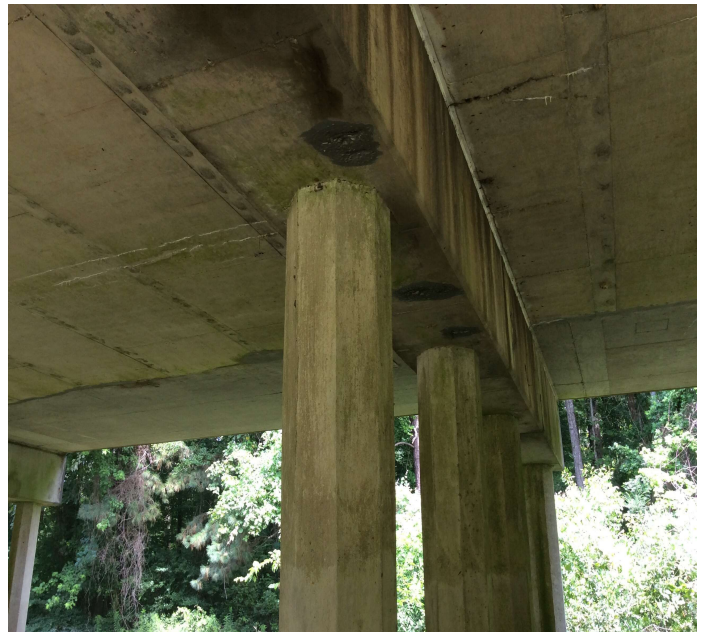
PHOTO 22 Description Bent 20 spalls on cap
