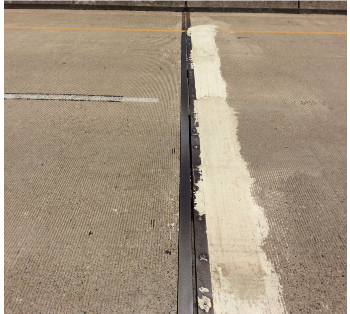
PHOTO 5 Description Pier 1 leaking/ missing 5 ft
