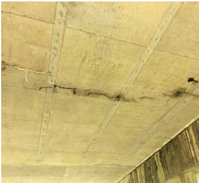
PHOTO 1 Description Span 13 bottom deck small delam With efflorescence staining . 36 sq ft total
