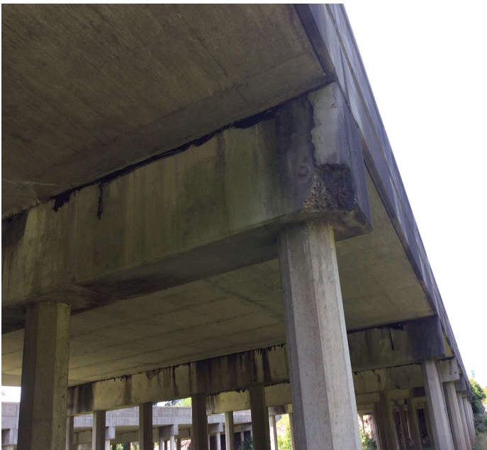
PHOTO 1 Description BT 8 lt end cap spall rebar exposed
