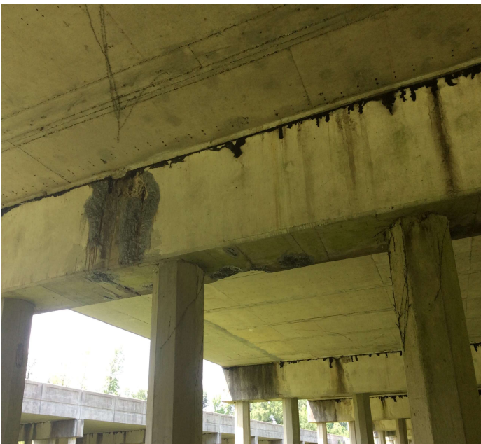
PHOTO 8 Description BT 11 spalls rebar exposed 10 LF
