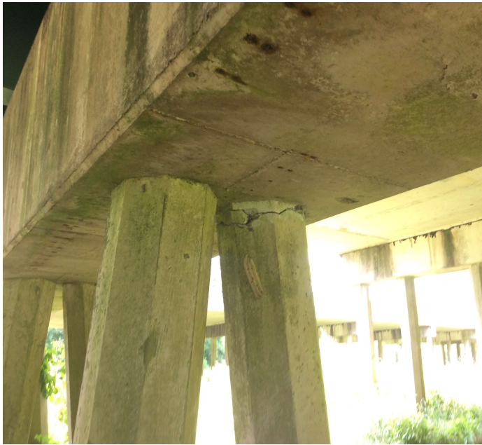
PHOTO 1 Description BT 15 main Spain pile 4 cracking in top of concrete pile
