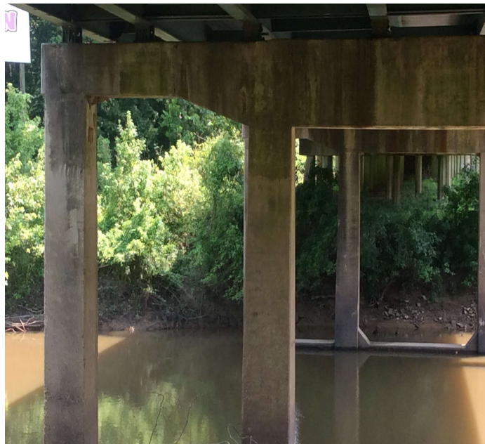
PHOTO 1 Description Pier 1 in water spall with rebar exposed 1 sq ft On It side at column 2
