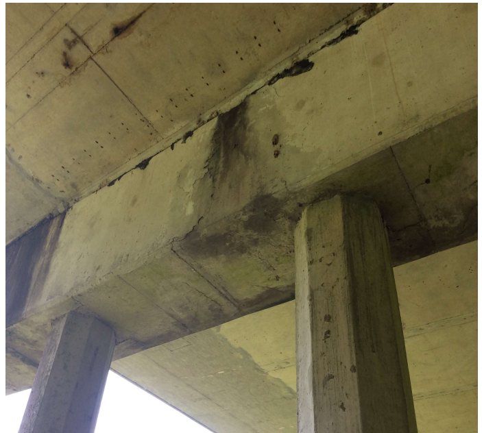
PHOTO 14 Description BT 5 delam on cap at pile 5&6 on cap 1 LF
