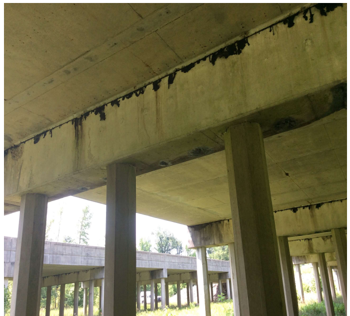
PHOTO 10 Description BT 9 cap spalls and rebar total 9 LF . 6 LF rebar exposed 2 LF delam
