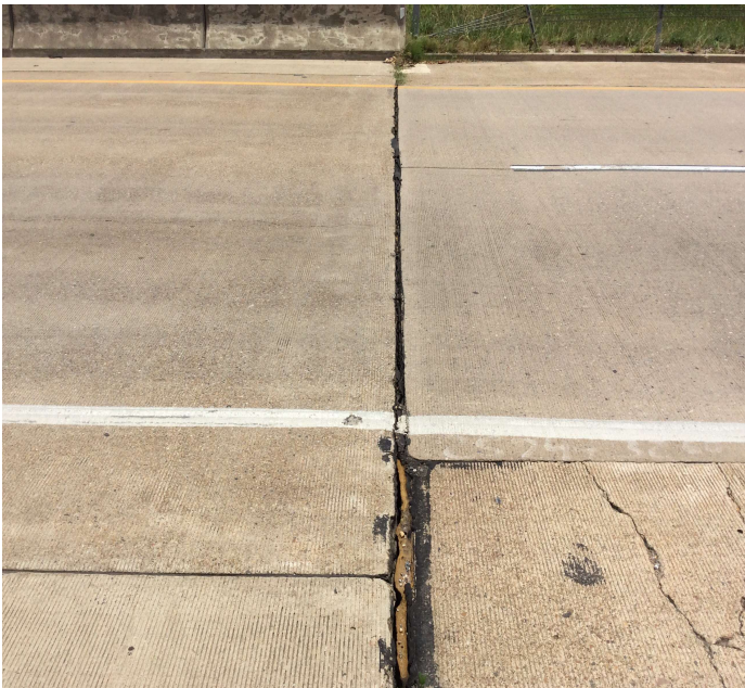
PHOTO 1 Description Bent 1 joint missing material
