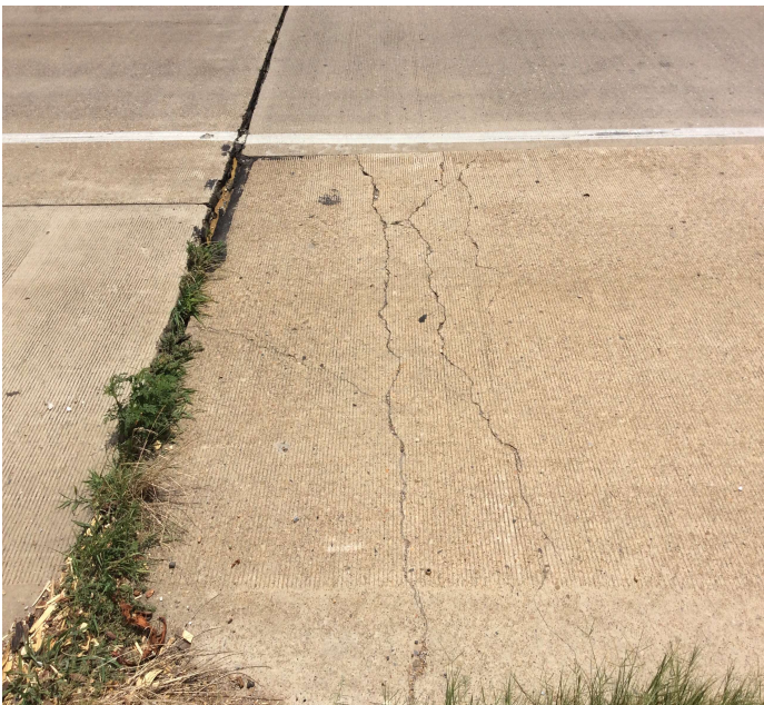
PHOTO 1 Description Bent 1 approach gutter cracks
