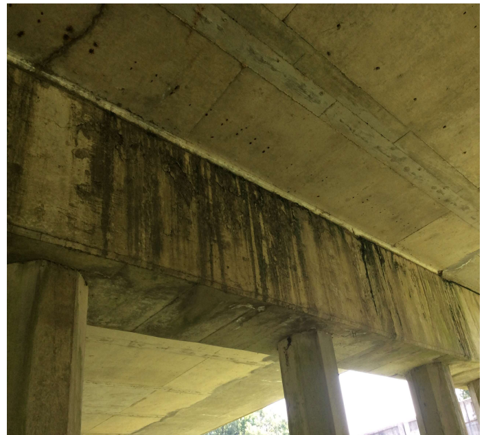
PHOTO 6 Description BT 14 spalls less than 1" depth 12 LF total
