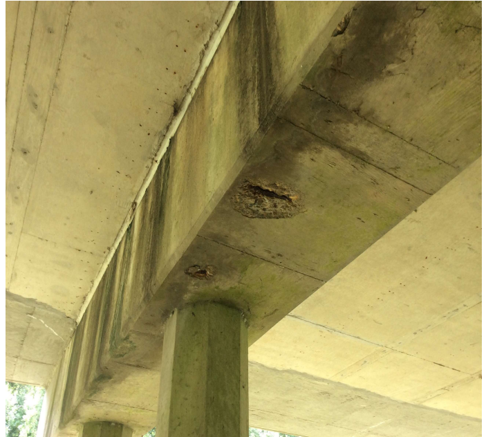
PHOTO 25 Description Bent 23 spalls rebar exposed
