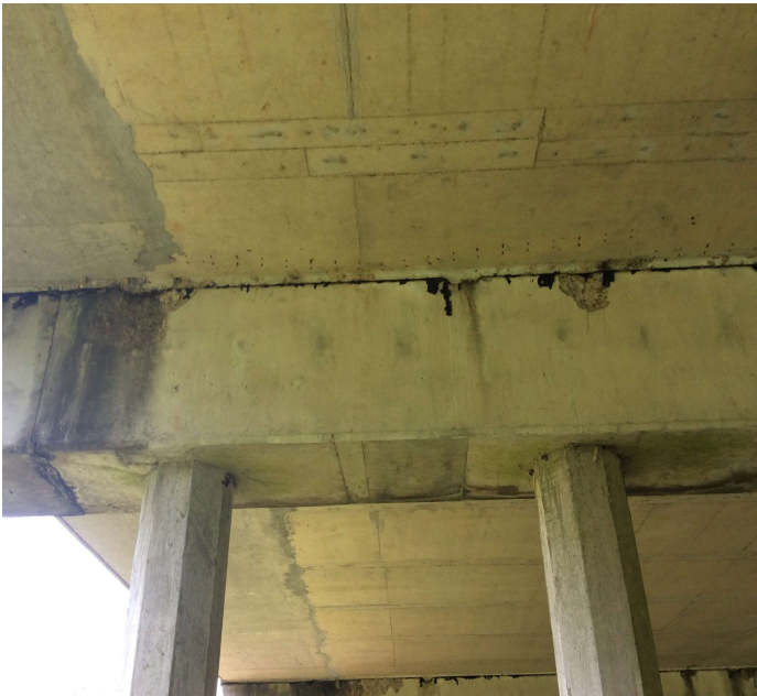
PHOTO 16 Description BT 3 cap spalls 3 LF
