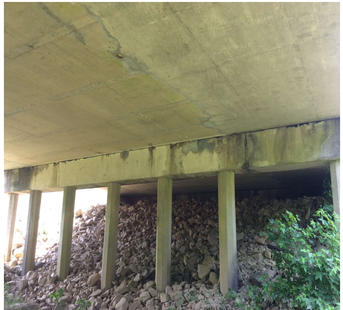
PHOTO 17 Description BT 2 cap spalled and some rebar exposed Spall 10 LF Rebar exposed 3
