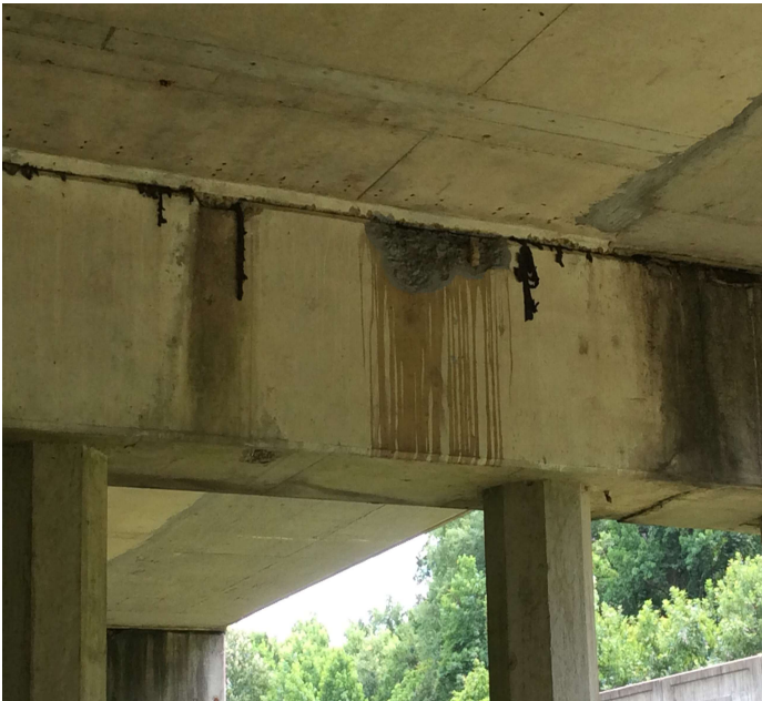
PHOTO 24 Description Bent 22 spall west face
