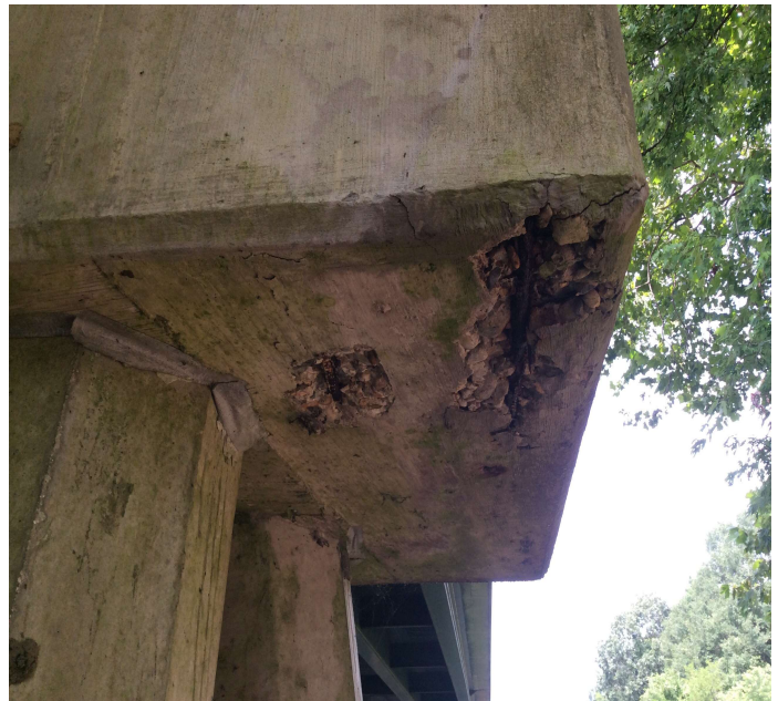
PHOTO 18 Description Bent 16 spall rebar exposed, bottom of cap, north end.
