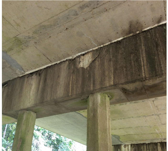
PHOTO 21 Description Bent 19 delamn on west face,small spall with rebar exposed on east face south end
