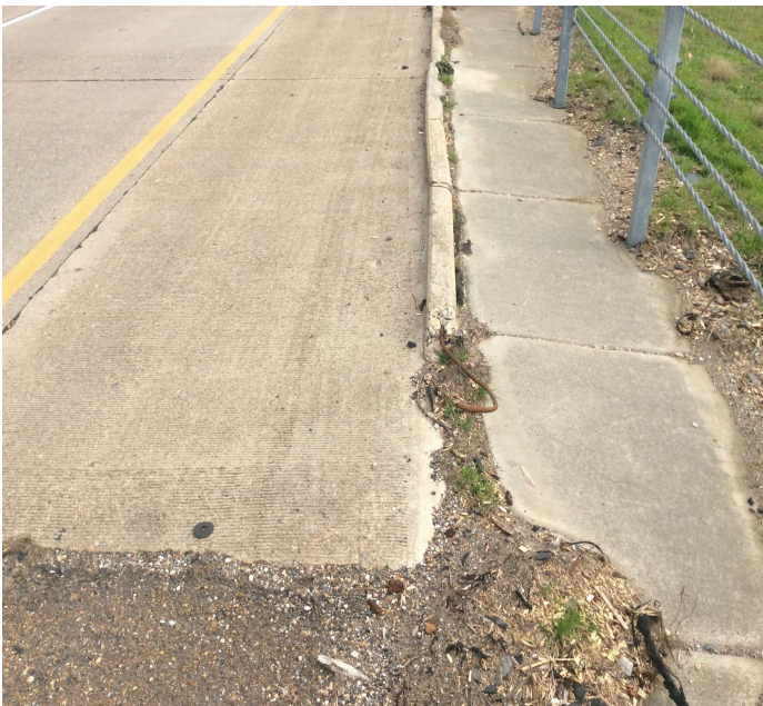
PHOTO 1 Description WHEEL GUARD BROKEN WITH REBAR EXPOSED 15 ft.
