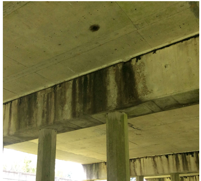
PHOTO 5 Description Bt 14 cracking 9 LF
