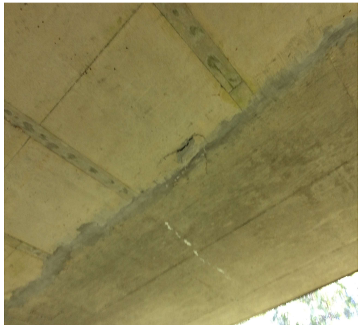
PHOTO 2 Description Span 7 delam 4 sq ft
