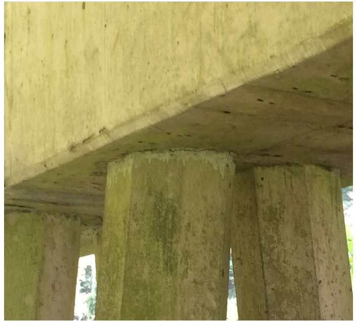
PHOTO 2 Description BT 15 main Spain pile 3 cracking in top of concrete pile
