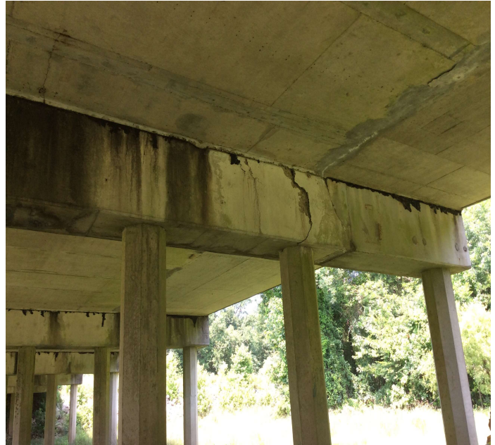
PHOTO 13 Description Bt 6 lt side delam at pile 2 on cap 2 LF Rebar exposed 2 LF on cap also.
