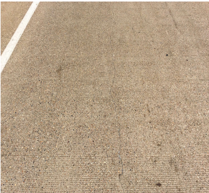
PHOTO 1 Description Sealable deck cracks all spans
