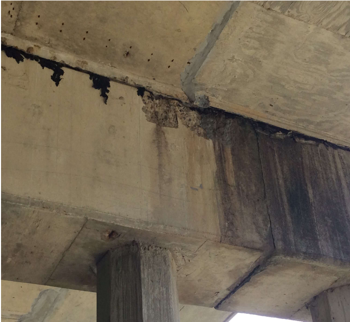
PHOTO 19 Description Bent 17 spalls top of cap west face south end
