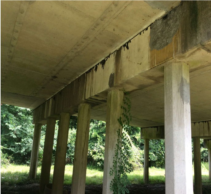
PHOTO 23 Description Bent 21 spalls and spalls with rebar exposed
