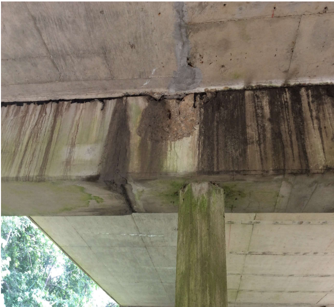
PHOTO 20 Description Bent 18 spalls with rebar exposed.
