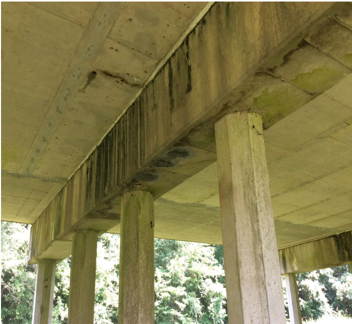
PHOTO 12 Description BT 7 spalls and delam total 6 LF Spall 2 LF Delam 4 LF
