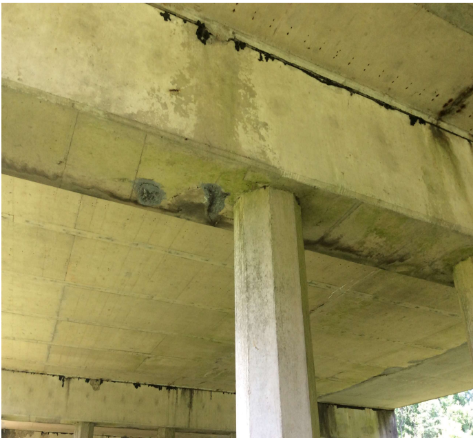
PHOTO 15 Description BT 4 cap 2 LF rebar exposed 1 LF delam
