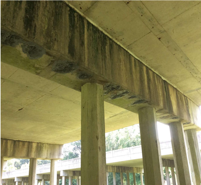
PHOTO 11 Description BT 8 spalls rebar exposed 13 LF total
